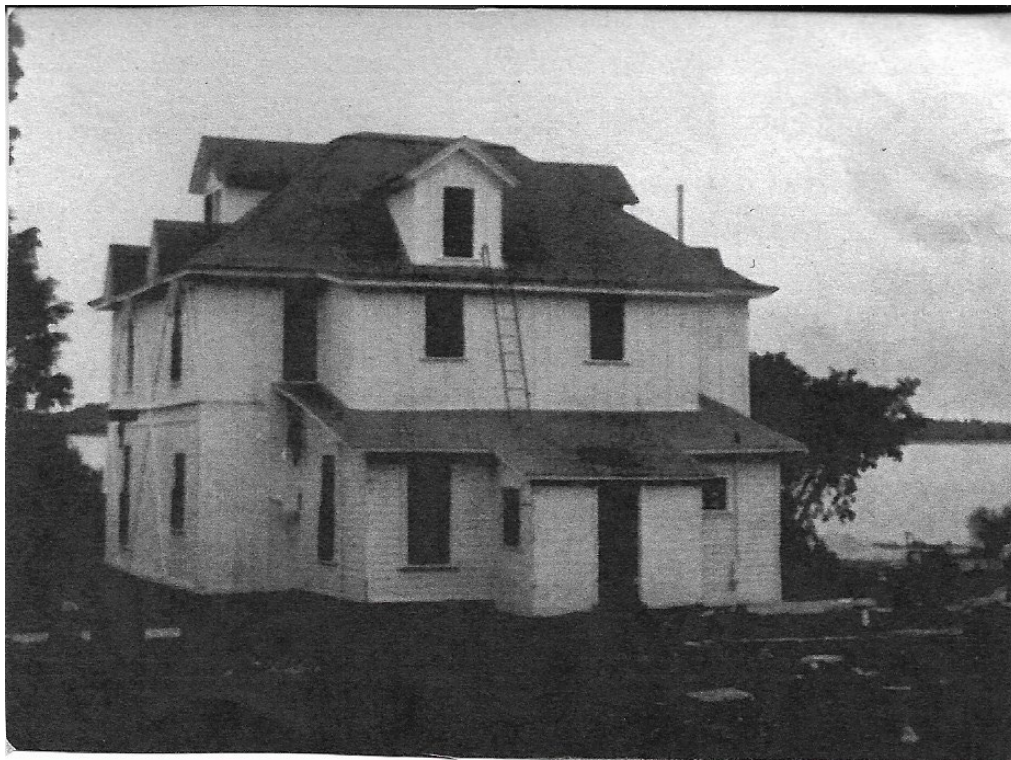
Rear elevation of cottage.
