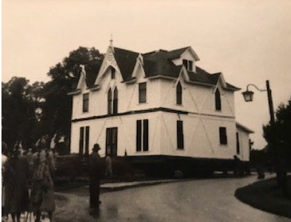
Cottage in process of move.
