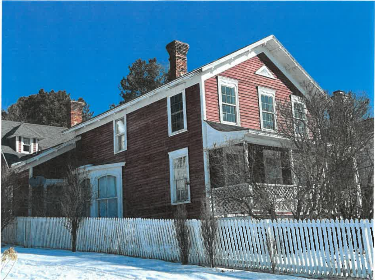
Photo 2. 6948 Main Street, c. 1850.
