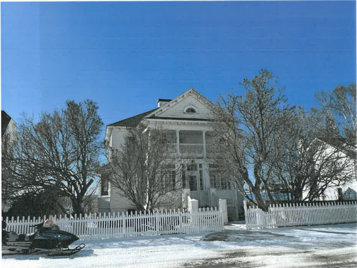
Photo 5. Saint Anne's Rectory, 6837 Main Street
