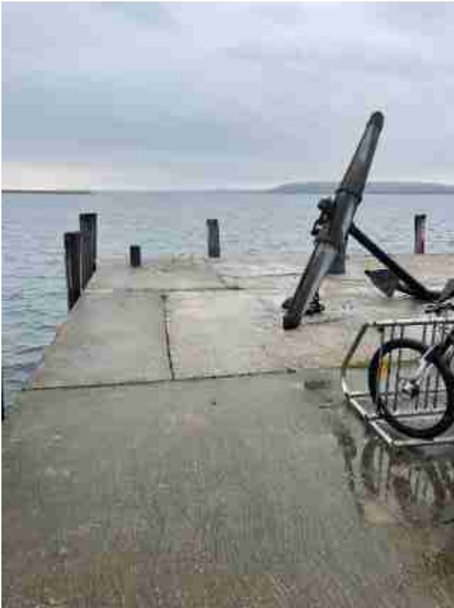
130) Deck (east end)
