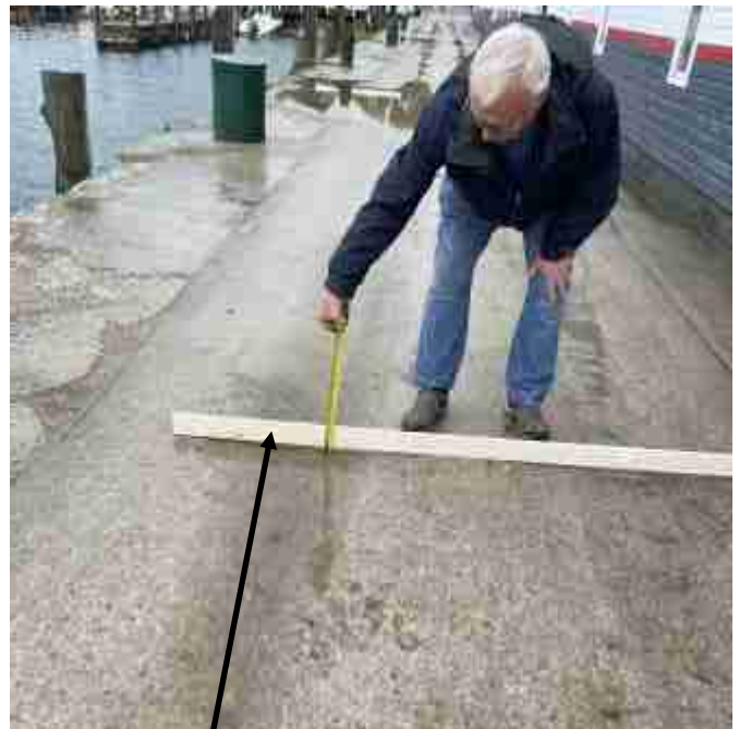
113) South deck area Apron metal 1 1/2' deck ware
