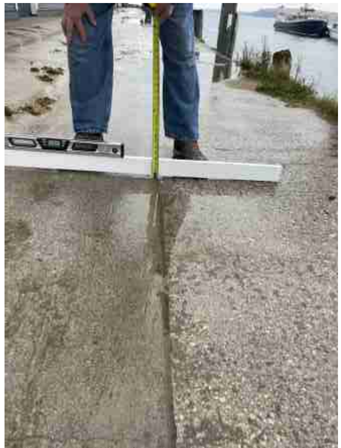
111) South deck area
