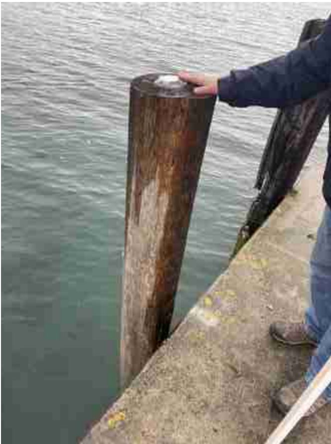
136) Bumper pile (north side)
