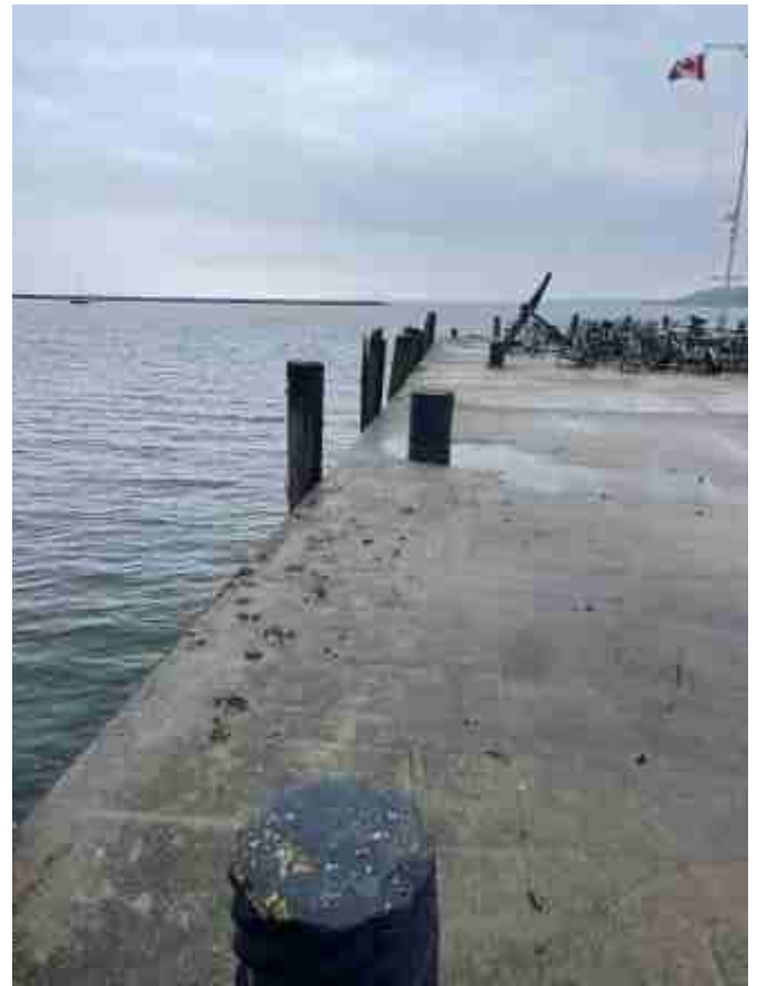
137) Bumper pile (north side)
