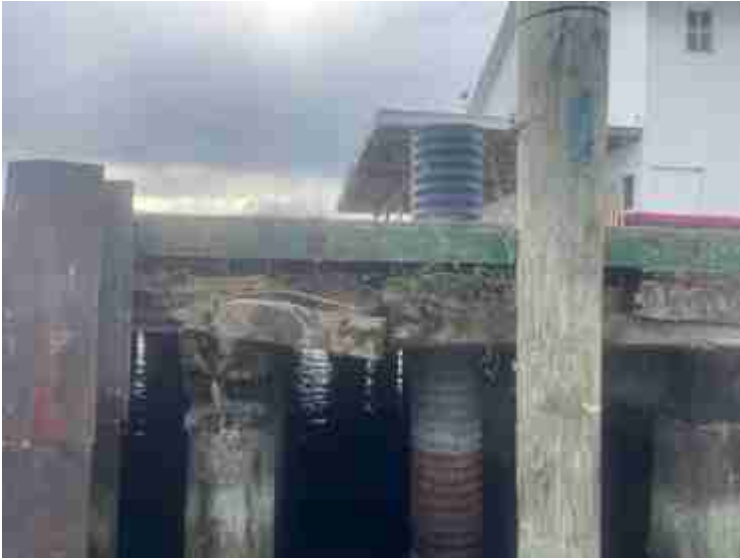
61) North dock at warehouse
