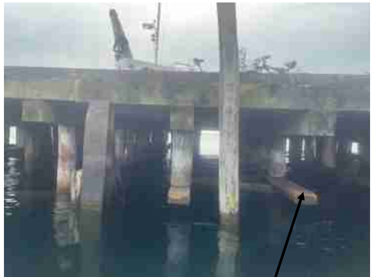
52) North dock east end
