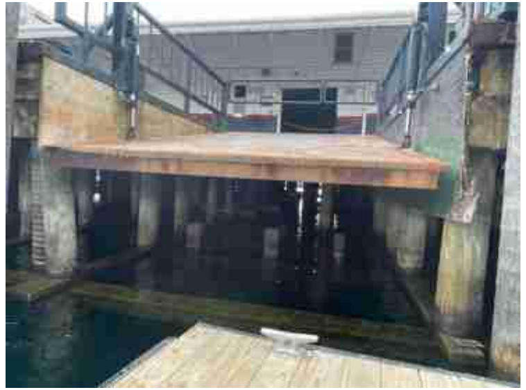
74) Dock (north) ramp (west end)
