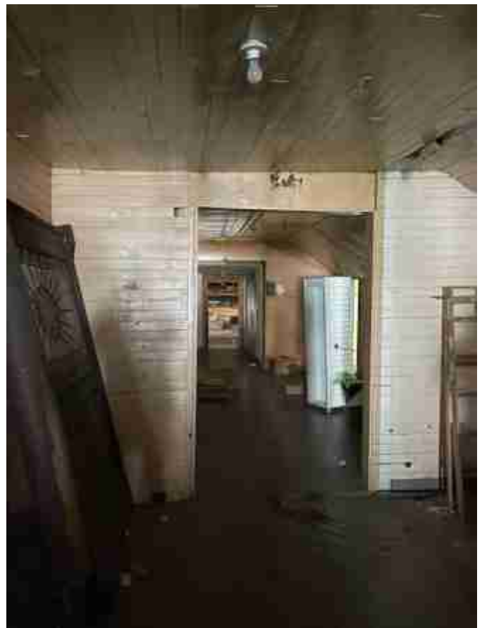
146) Lower level of warehouse
