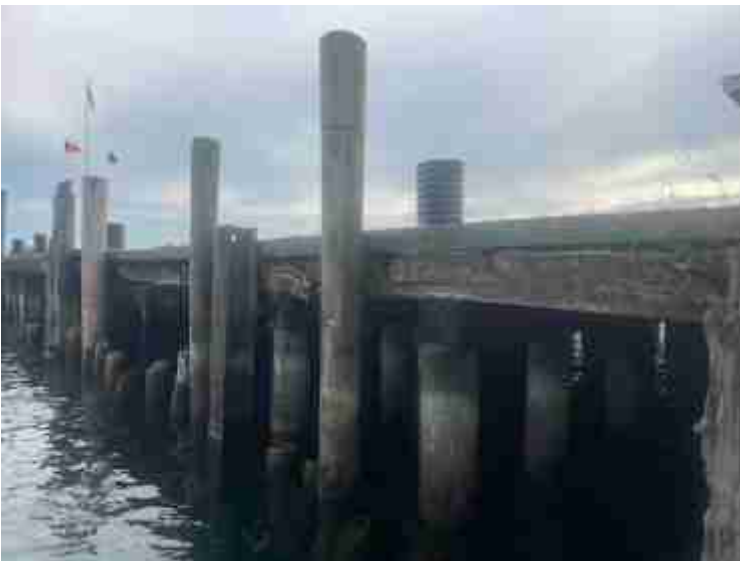
63) North dock at warehouse looking east
