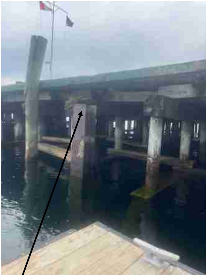
Horizontal bracing removed 55) North side east end
