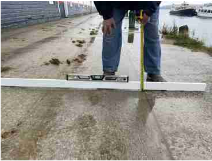
110) South deck area
