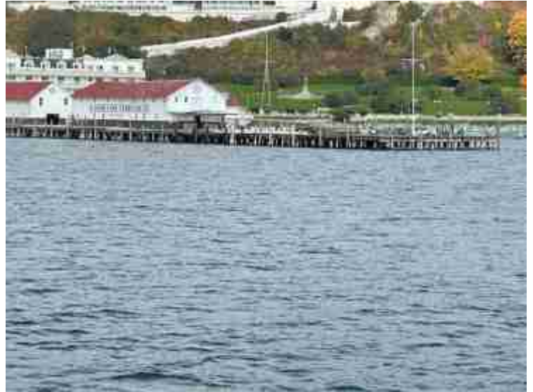
2) South side of dock at east end
