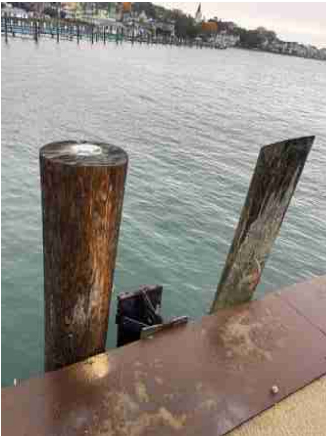
139) Reinforced deck (north side)
