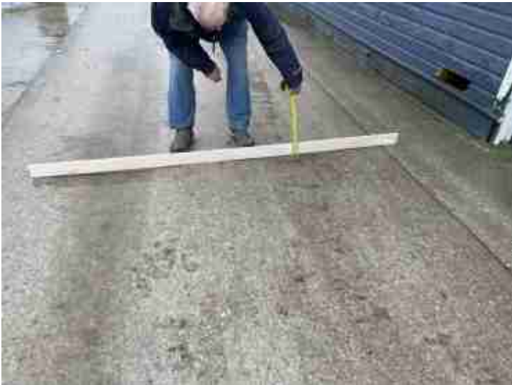
112) South deck area
