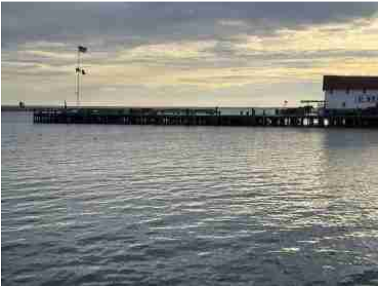
96) North side (east)
