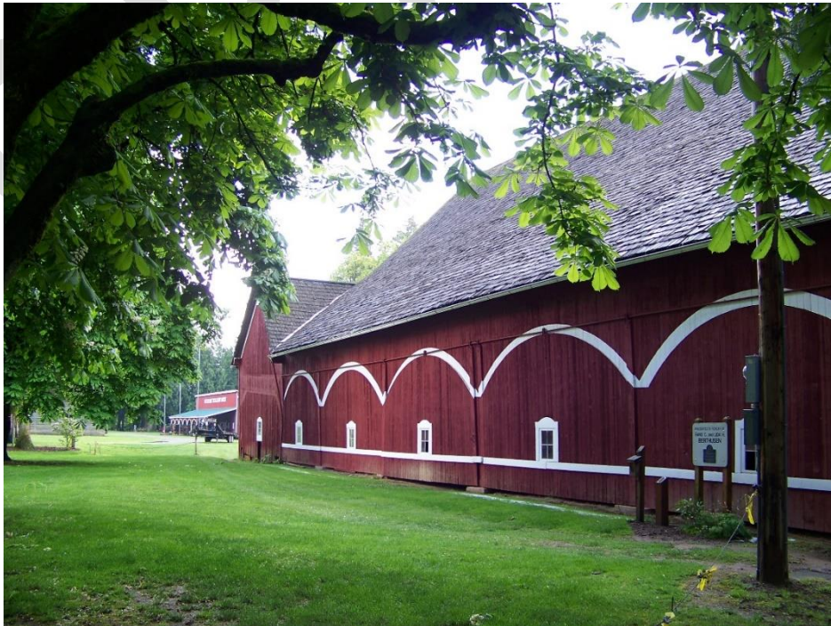
The historic Berthusen Barn built in 1901
