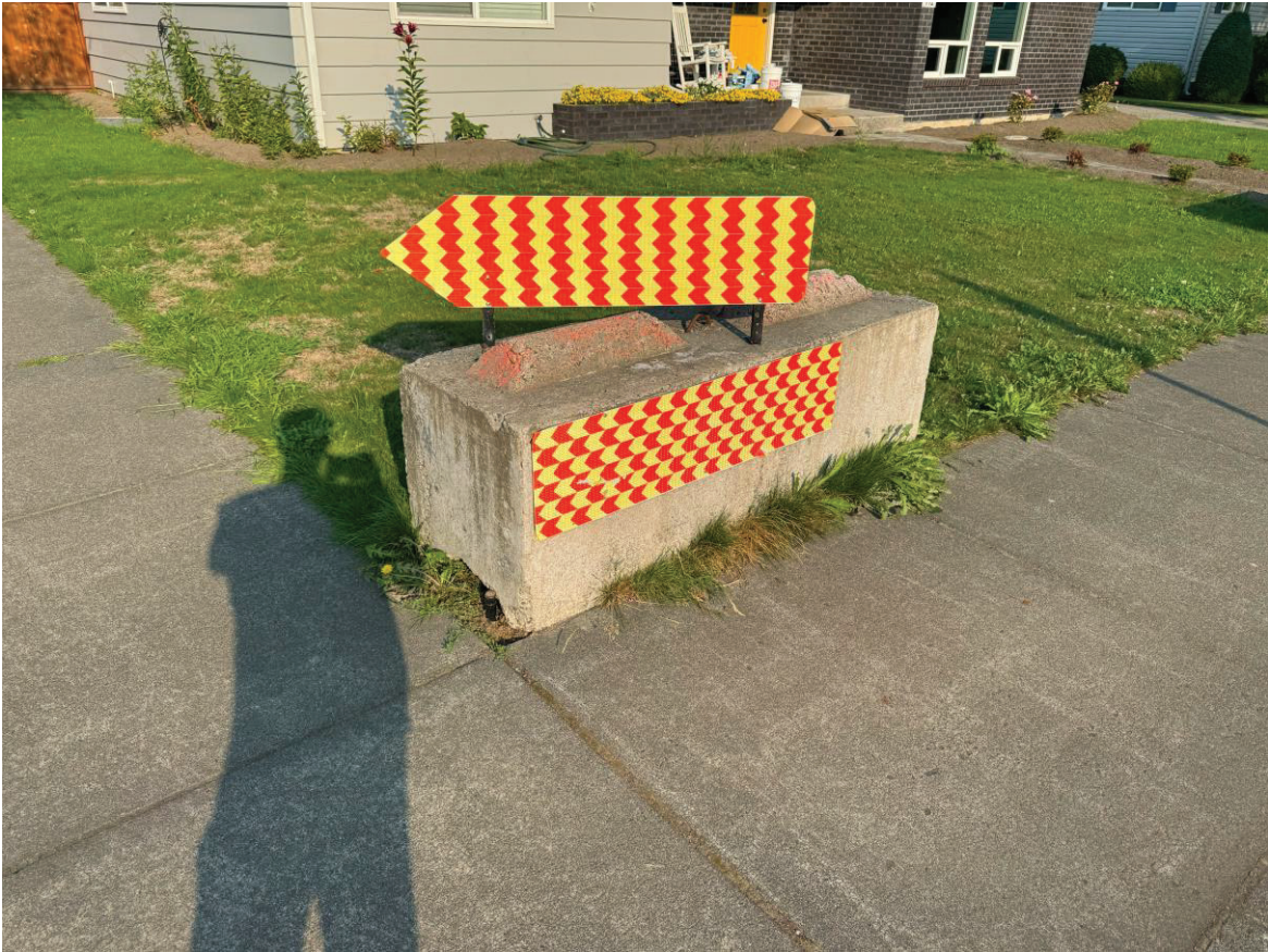
Figure 2 Example of Concrete Block and Turn Arrow Located at Intersection
