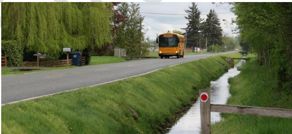
Pepin Creek flowing directly adjacent to Double Ditch Road in Lynden.
