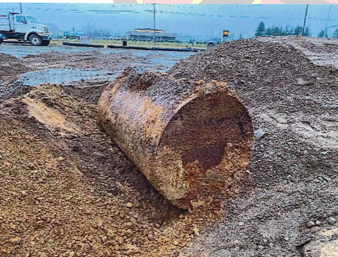
Fuel tank inspection new Shell station discovery
