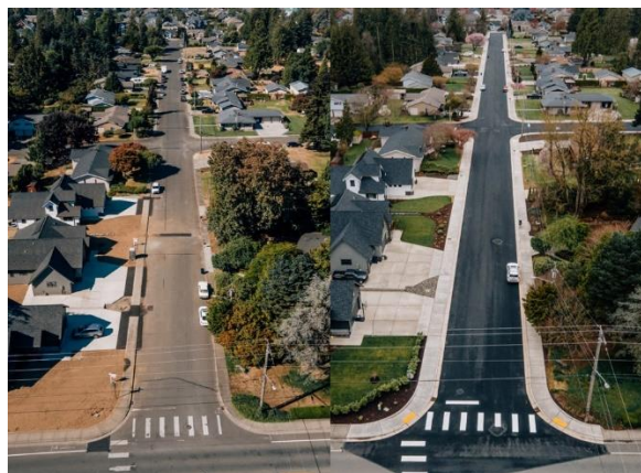
South Park Waterline & Overlay (Before & After)
