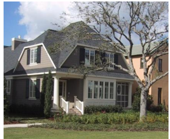
Above: Small-lot single-family home with alley access that fronts on a park.
