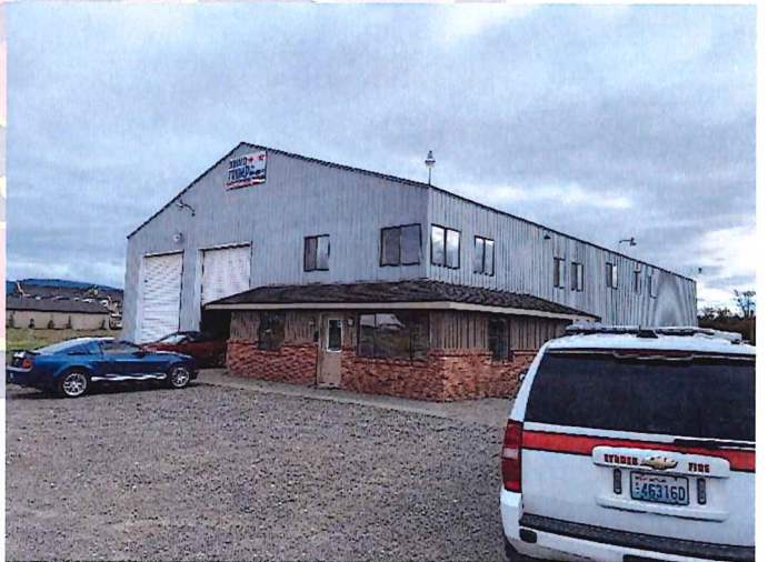
Temporary station at 1205 E. Badger
