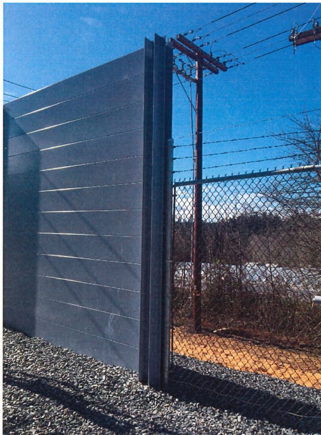
Figure 2: Proposed 9 ft. Non-conductive solid fencing and 7 ft. chain-link fencing with barbwire on top
