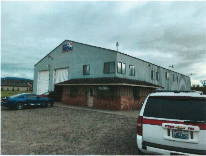
Temporary fire station
