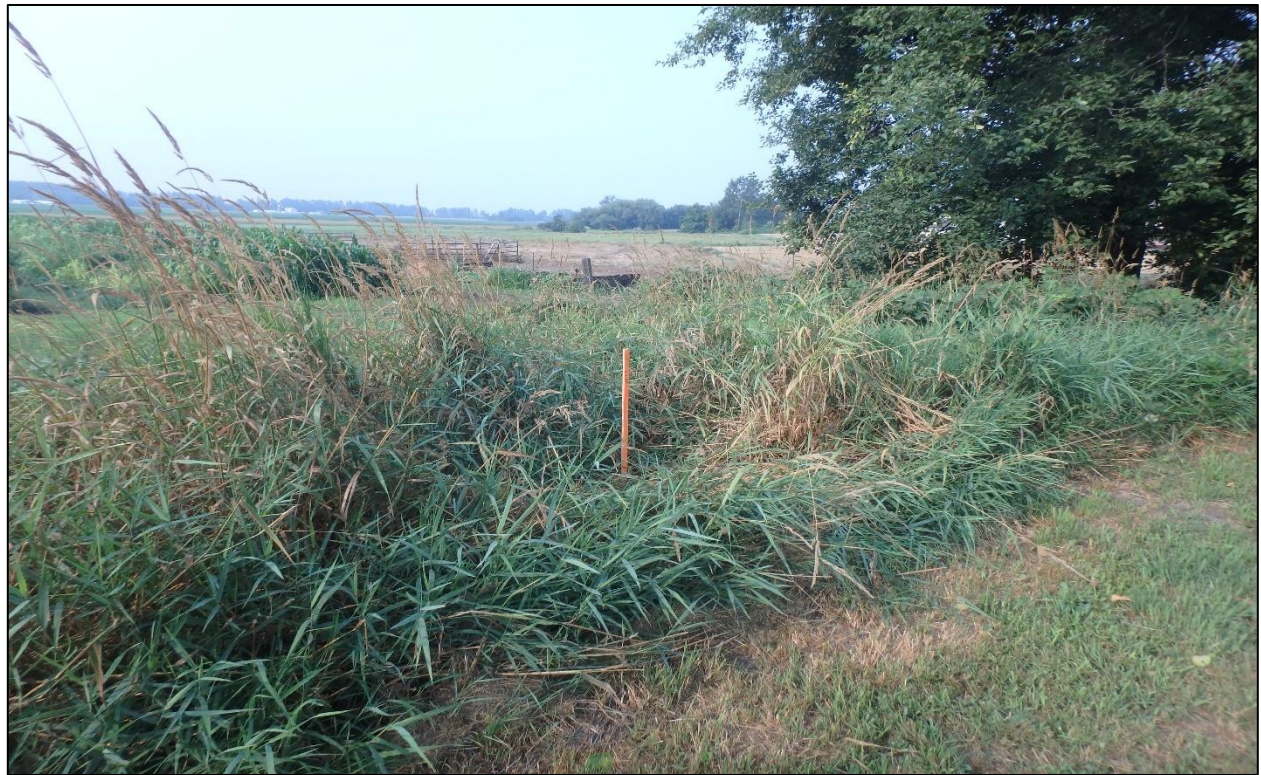
Photo 3. Overview of the Kamm Creek diversion / irrigation ditch, view to the southwest, towards the Sewer Line tie-in. Note the staked centerline.
