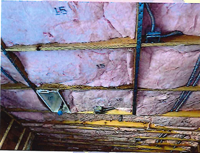
Downstairs ceiling insulation
