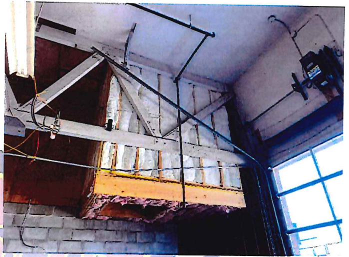
Fire pole enclosure
