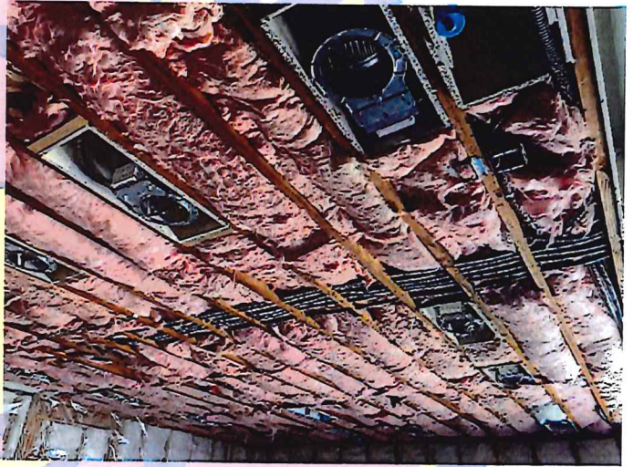
Kitchen insulation and can lights
