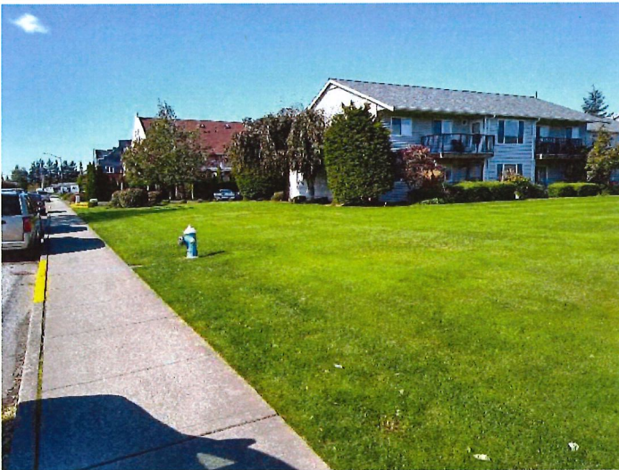
Existing Parkview West Apartments
