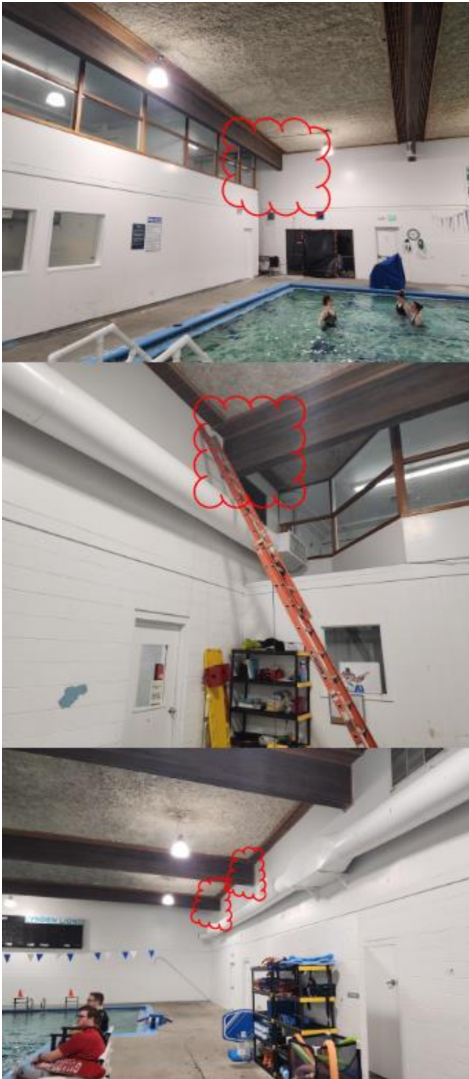
Figure 2: Location of moisture content testing on glulam beams.
