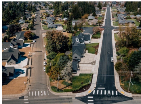
South Park Waterline & Overlay (Before & After)
