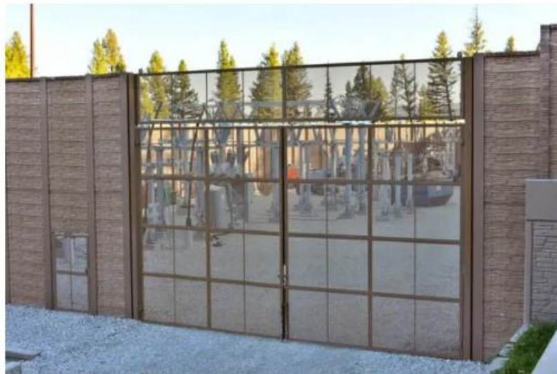
Drive gate for Big Sky, Montana, Substation project, plus Superior Cobblestone™ screening wall from Superior Concrete Products.
