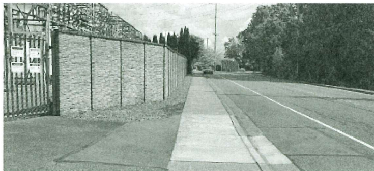
Figure 1: Existing 8 ft. concrete paneling fencing along E. Front Street at Lynden Substation
