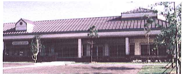
Uninteresting Roof Line Individuality of the stores is lost.
