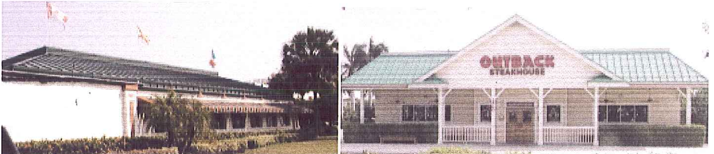
The roofs on these structures are examples of Hip on Deck roof styles.
