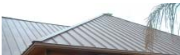
Standing Seam Sheet Metal
