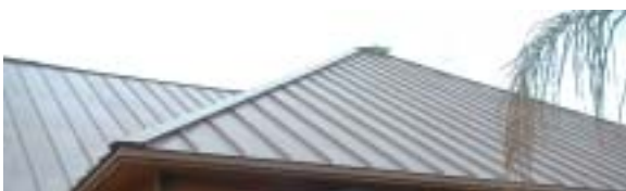
Standing Seam Sheet Metal
