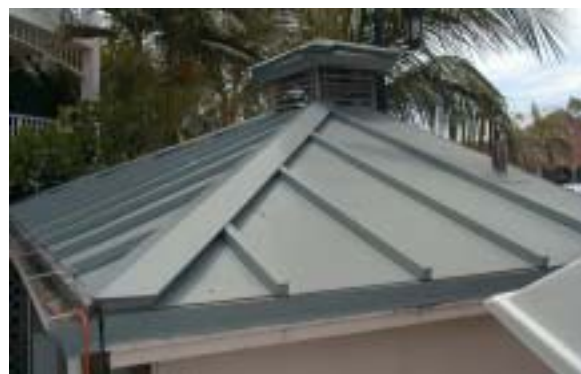
Standing Seam Sheet Metal
