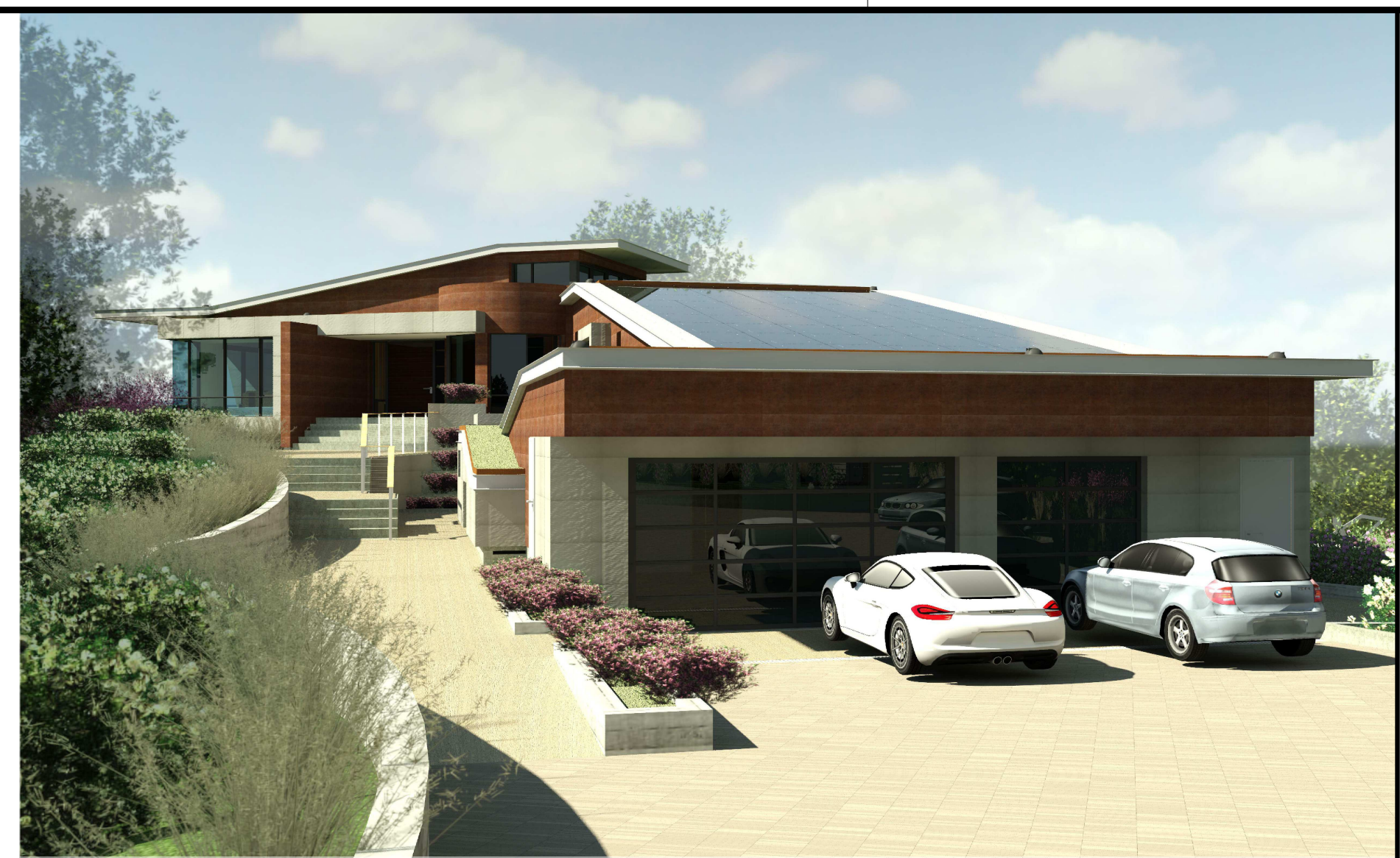
VIEW FROM DRIVEWAY
