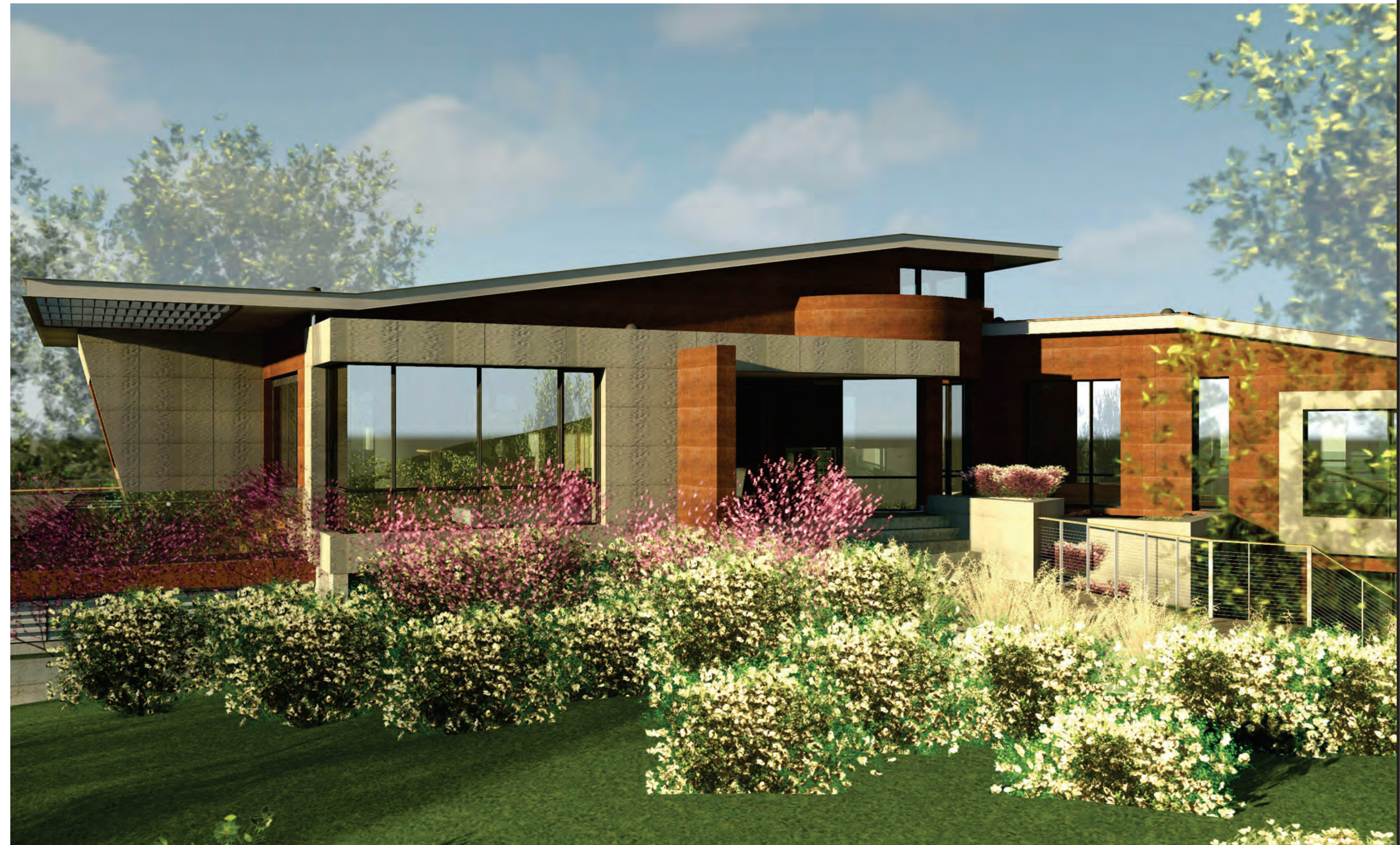
VIEW TOWARDS FRONT ENTRY
