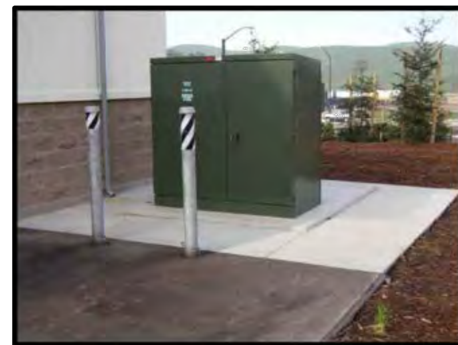
PG&E PAD MOUNTED IIE 3Ø TRANSFORMER PAD SIZE: 90"X106" CABINET SIZE: 89"W X 90"D X 77"H
