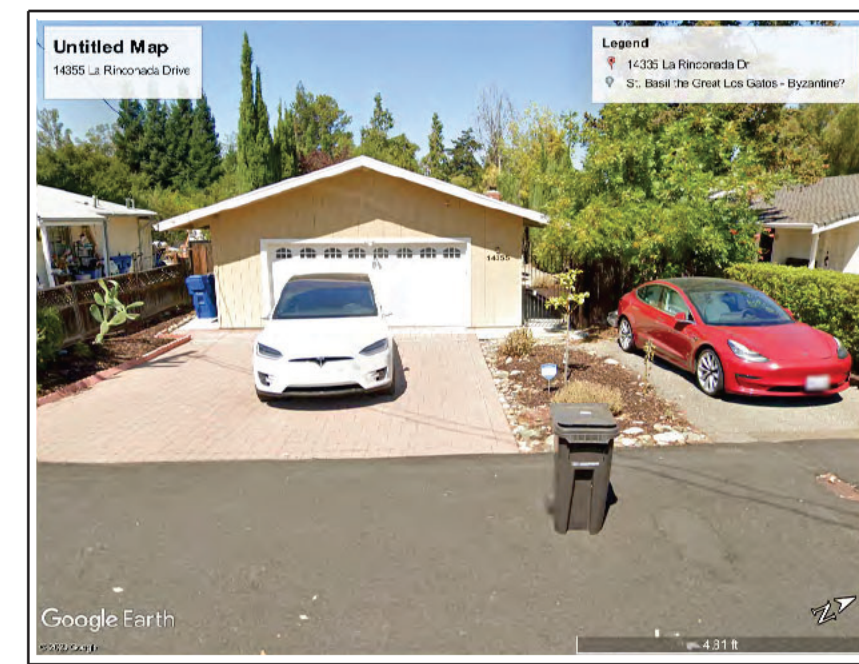
14355 La Rinconada Drive View - West
