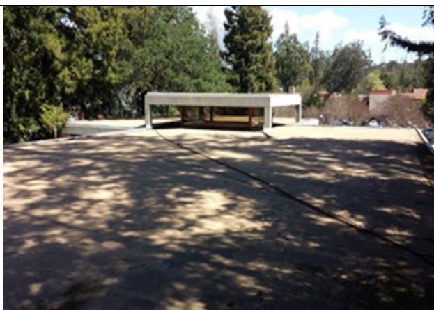
I Police Headquarters Roof Repair
