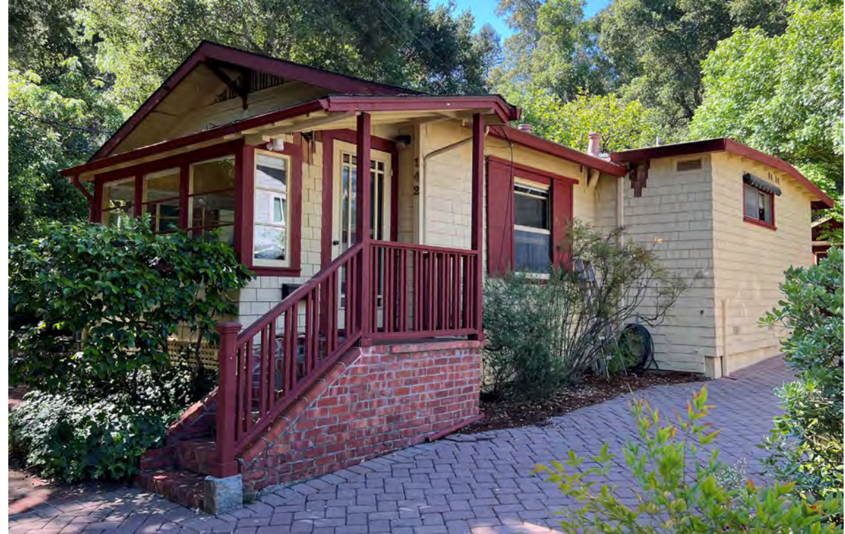
PORCH STAIR ADDITION
