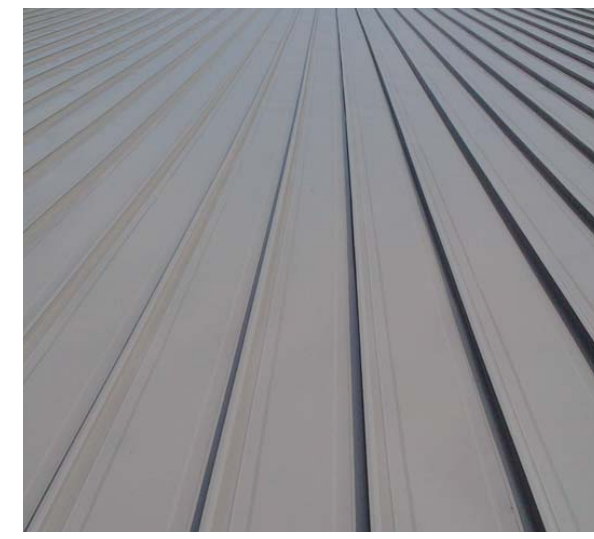
4 ROOF STANDING SEAM METAL
