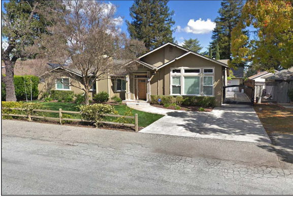
The Site and Existing House
