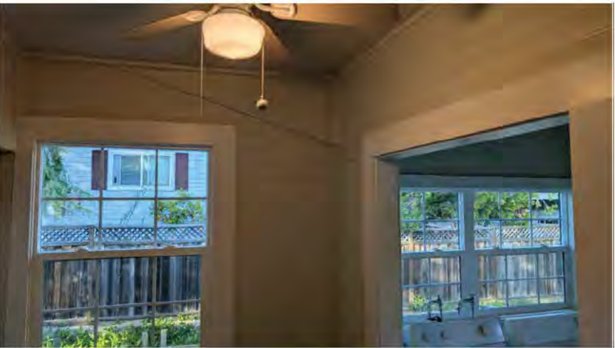
PHOTO 1 SHOWING OLD SLOPING ROOF PROFILE ON WINDOW SIDE
