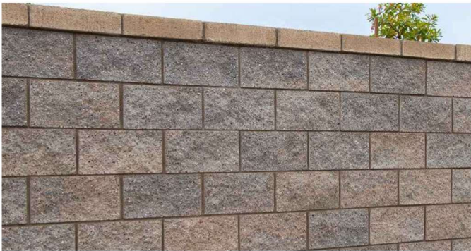
A RETAINING WALL SHALL BE VARIEGATED CMU WITH WALL CAP FROM ORCO BLOCK AND HARDSCAPE COLOR SHALL BE BORREGO SPLIT FACE ON EXPOSED SURFACE LRV SHALL BE MAX 30%
