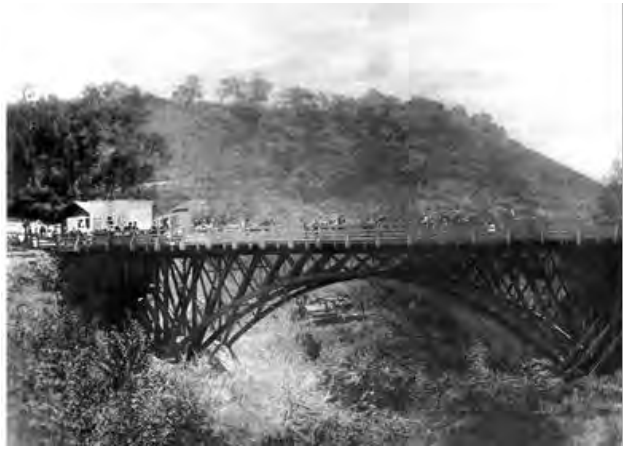
1900, Main Street Bridge
