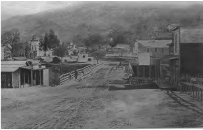
1890's Main St. Bridge
