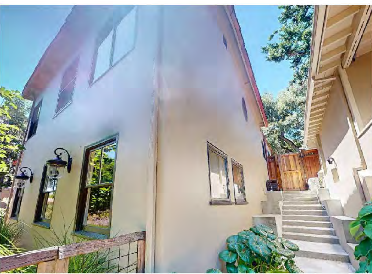
LEFT OF RESIDENCE - SHOWING REAR OF ACCESSORY BUILDING TO BE REMOVED
