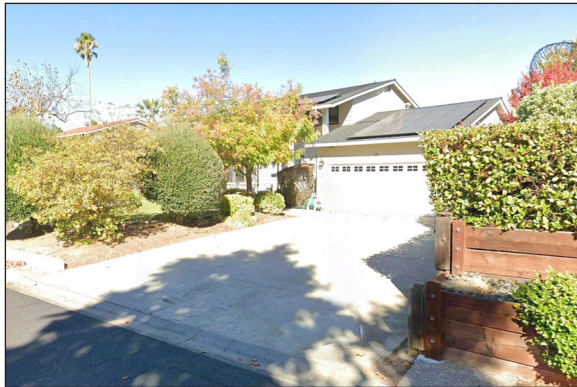
House immediately to the left
