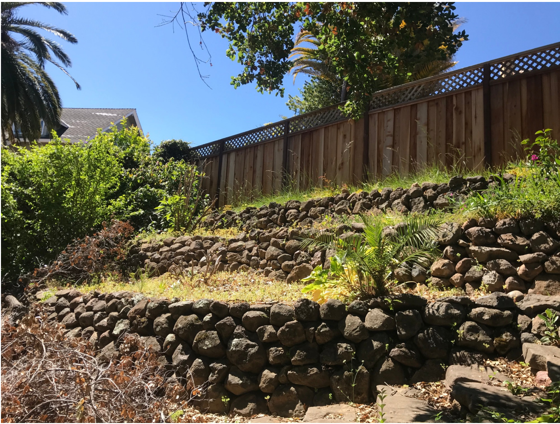
Left over retaining walls at rear yard
