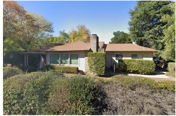
EXISTING HOUSE ON THE SITE: Hillow Road Facade
