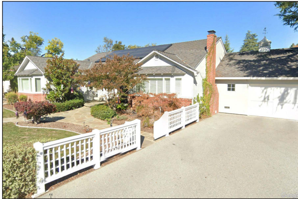
House immediately adjacent to the site on Hillow Road
