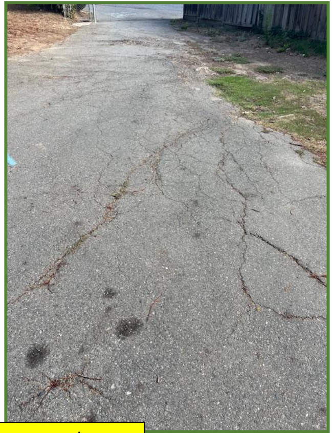
Hardscape damage due to extensive surface roots from Trees No. 947 & 948
