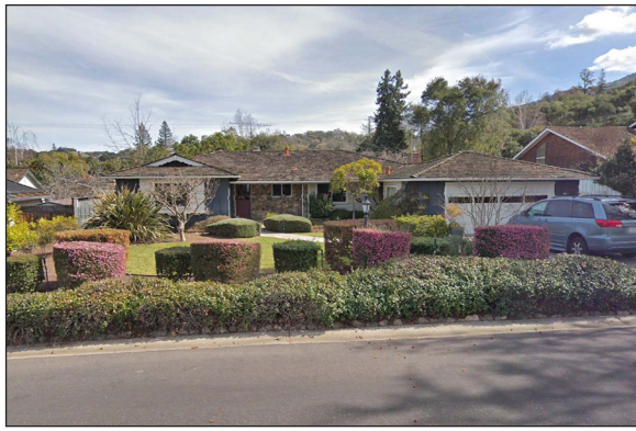
The Site and existing house
