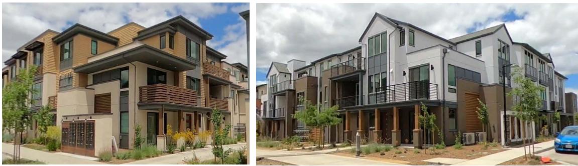
North 40 Phase 1 End Structures
