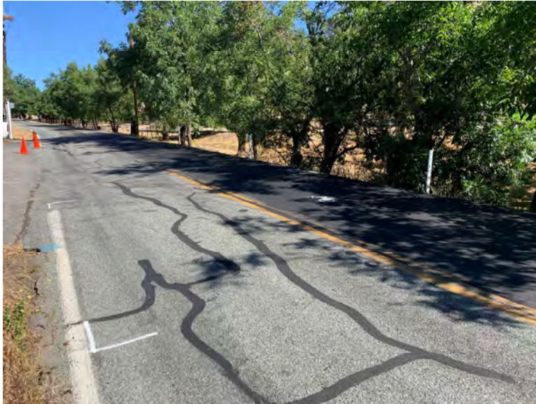
Road Condition at Boring B-1 (June 22, 2020)
