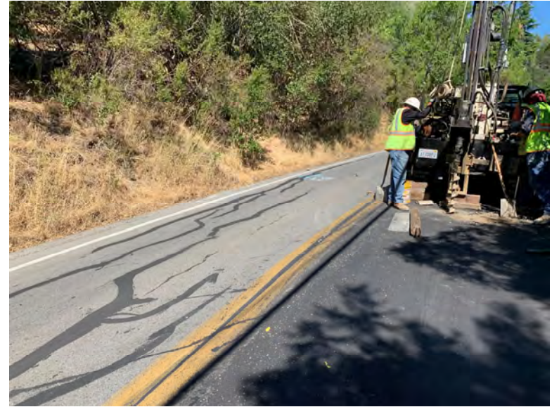
Road Condition During Drilling at Boring B-11 (July 1, 2020)
