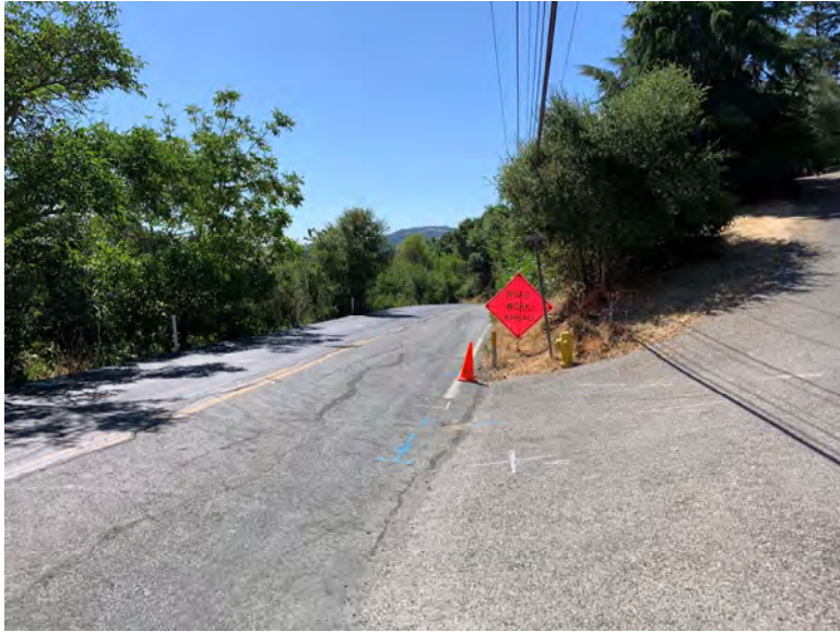
Road Condition at Boring B-12 (June 25, 2020)
