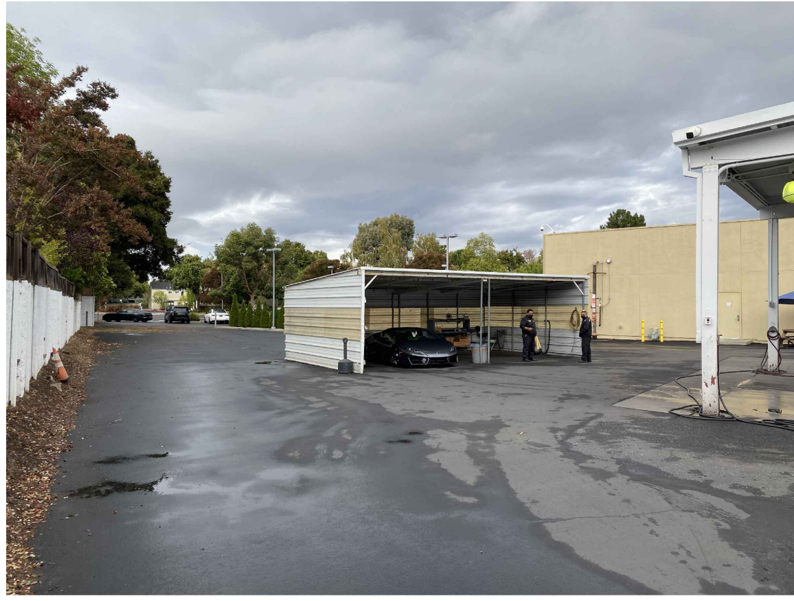
G. SOUTH LOOKING WEST
