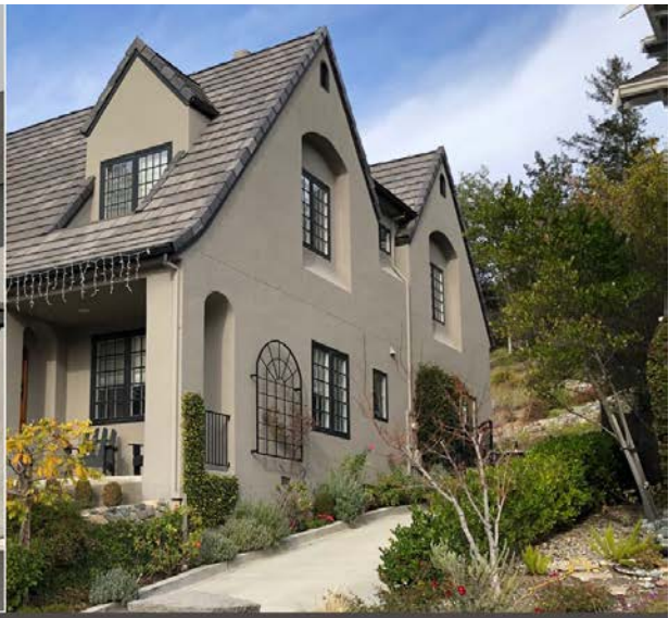
Existing Design Example 205 Loma Alta Avenue
