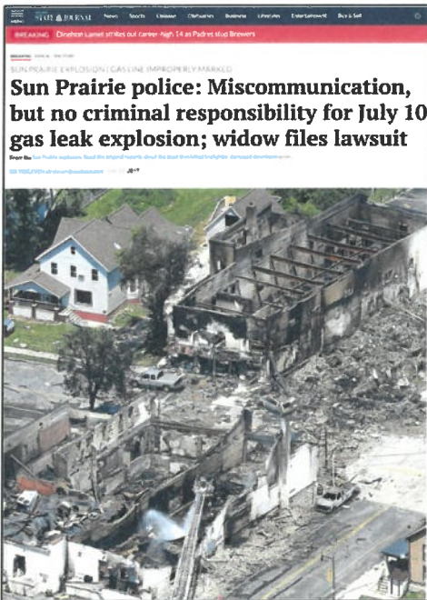
Accidents locating gas lines have severe consequences for contractors.
