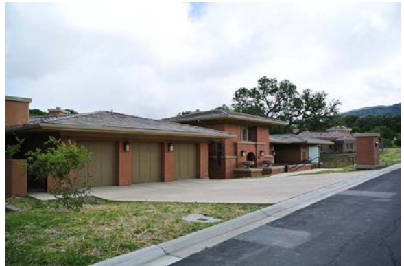
Nearby House on Santella Court
