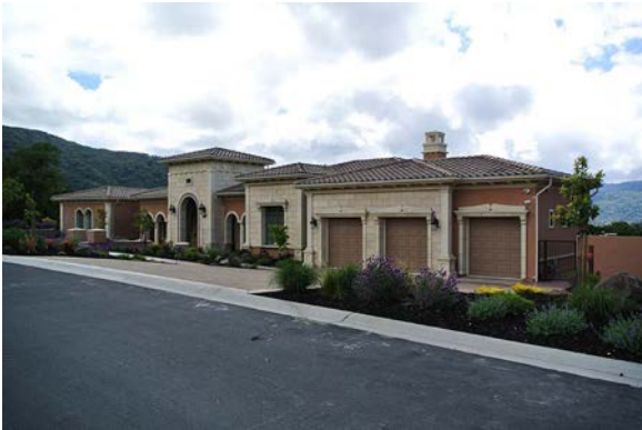
Nearby House on Santella Court
