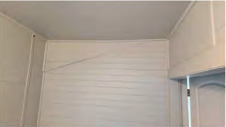
PHOTO 2 SHOWING OLD ROOF PROFILE ON BEDROOM 2 SIDE
