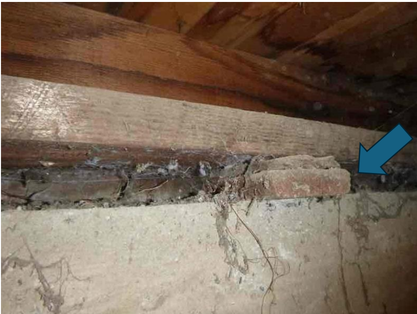
2B. Shimmed floor joists and mud sill
