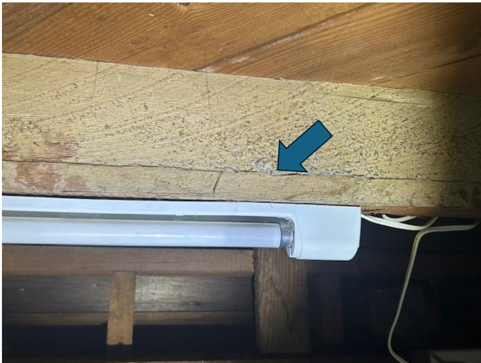
2C. Cracked 2x6 floor joists. Some spans are up to 9 feet.
