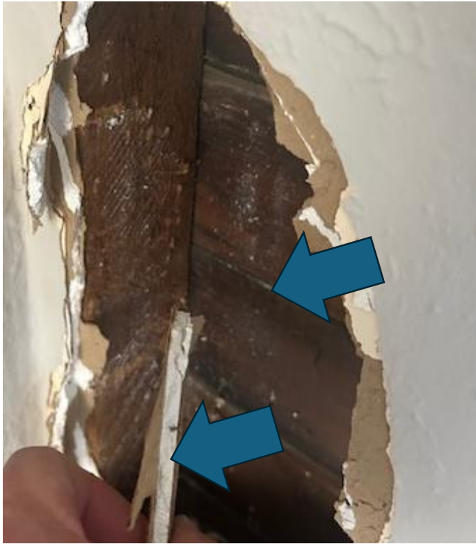
5D. Termite damage (rear door)
