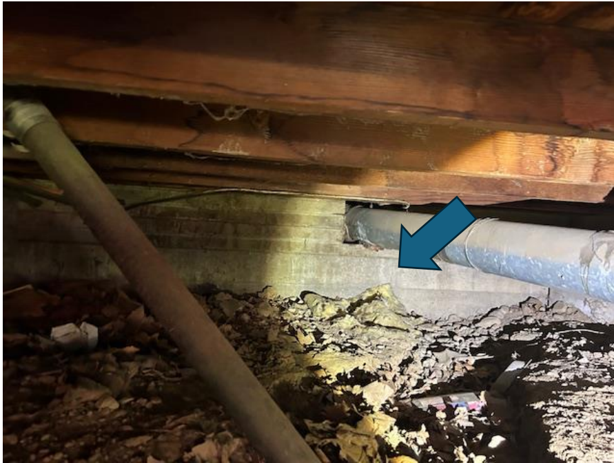
4B. Rear Addition – Original Exterior Foundation Wall
