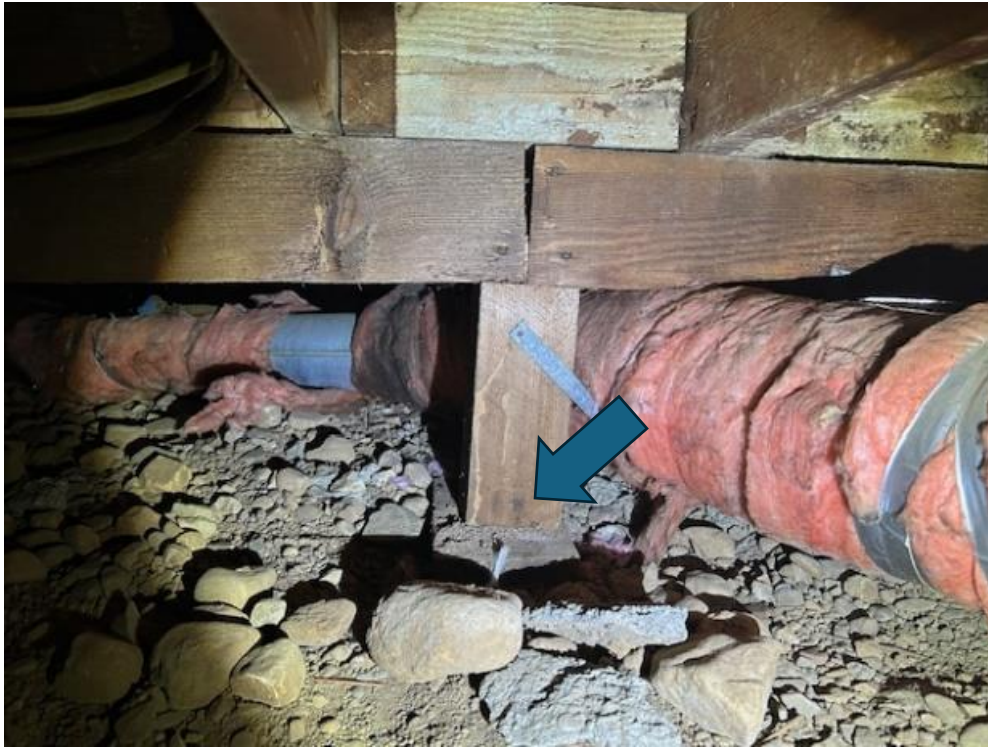
2D. Post framing against dirt.
