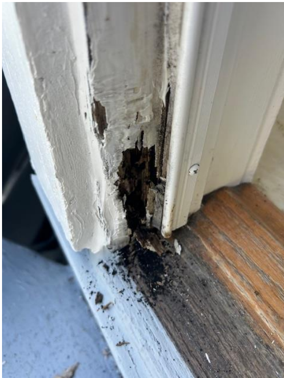
5D. Termite damage (rear door)
