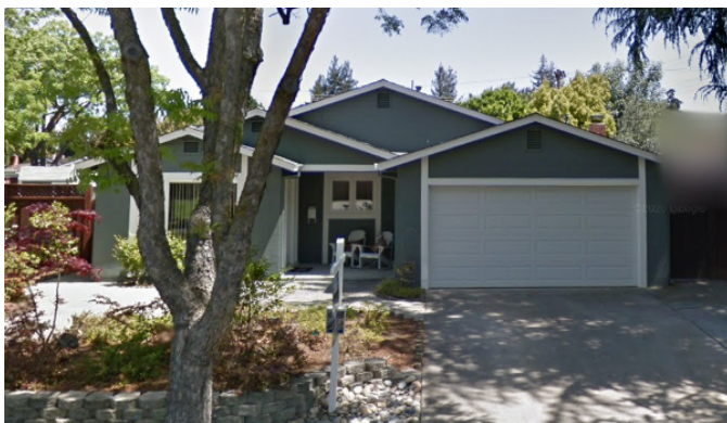
Gable Garage Roof at 143 Arroyo Grande Way (Across the street)
