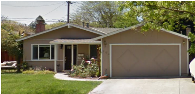
Gable Garage Roof at 144 Arroyo Grande Way (Immediate Left)
