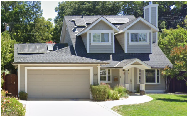
Two-story home at 209 Arroyo Grande Way
