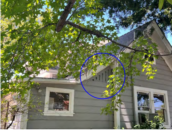
Image E, Pierced Balustrade Fretwork, Present Day
