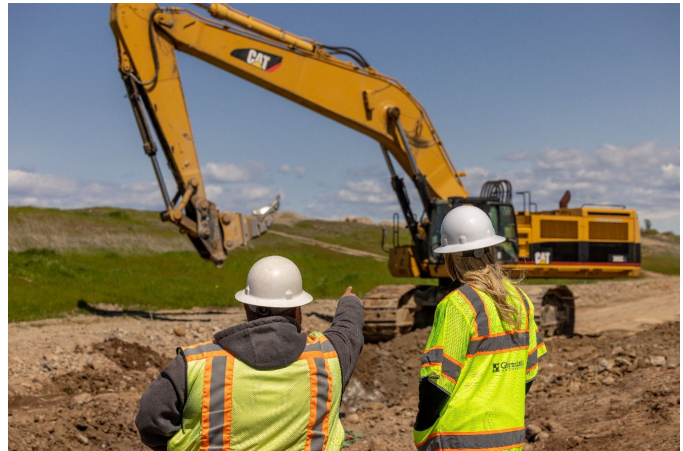
Inspection of Rough Grading, Bickford Ranch Development
